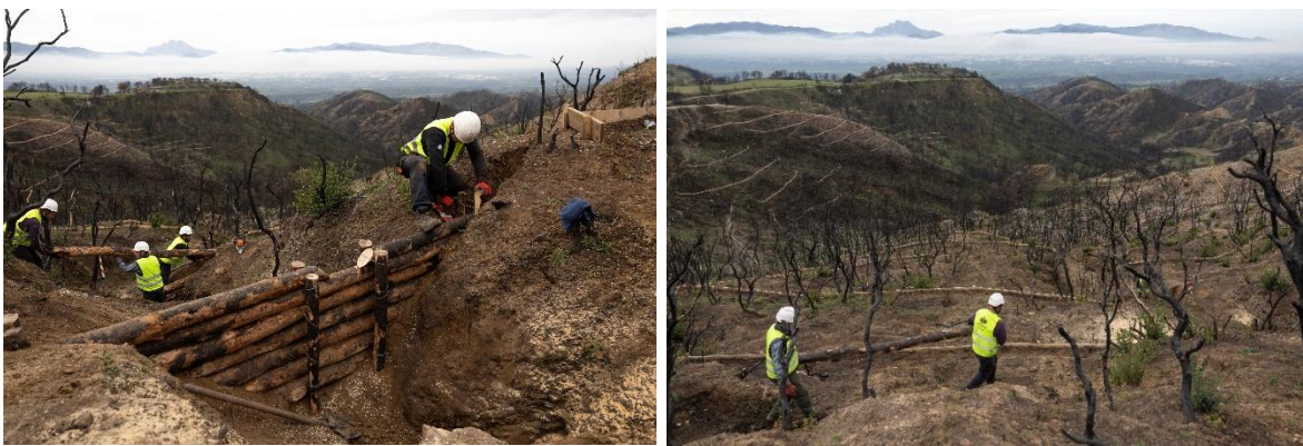
Achaia (Partas region, Greece) anti erosion and flood prevention
